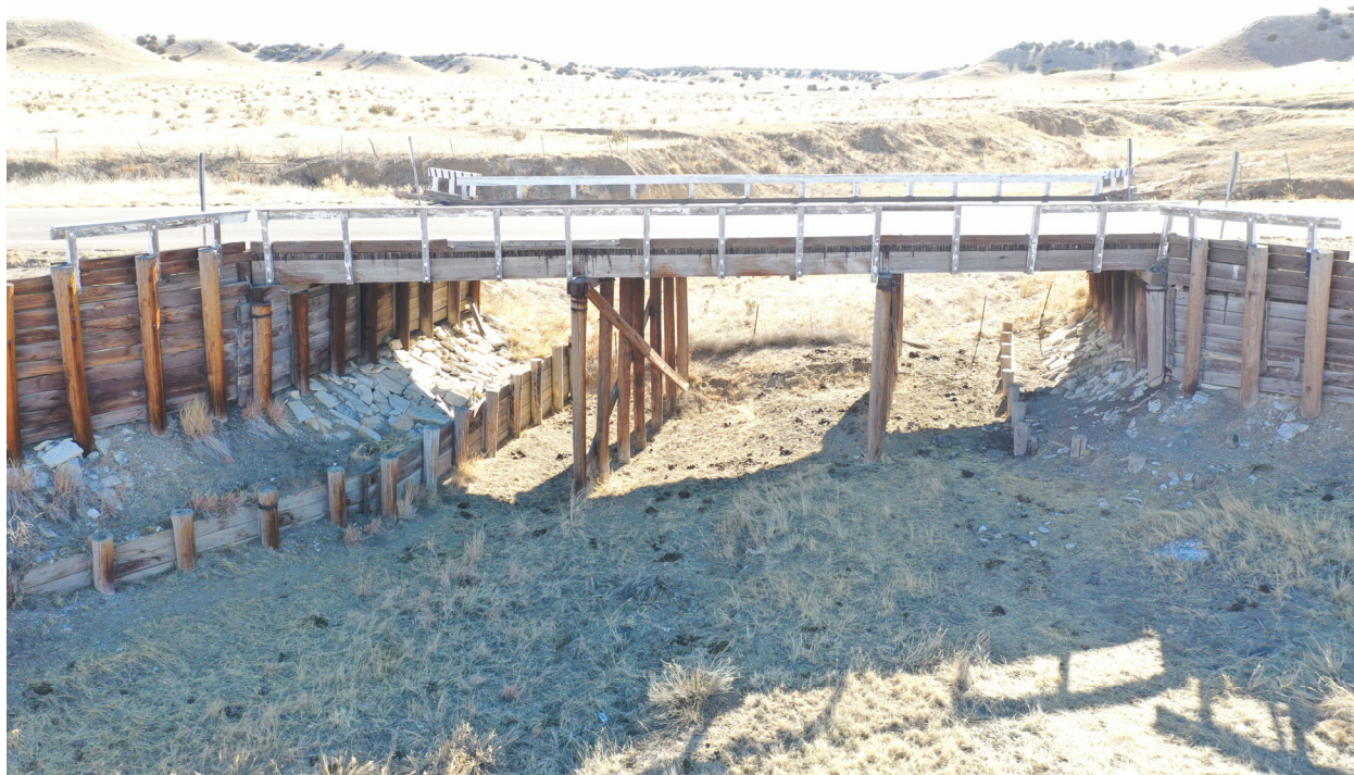
Picture 1 - Bridge N-21-C
