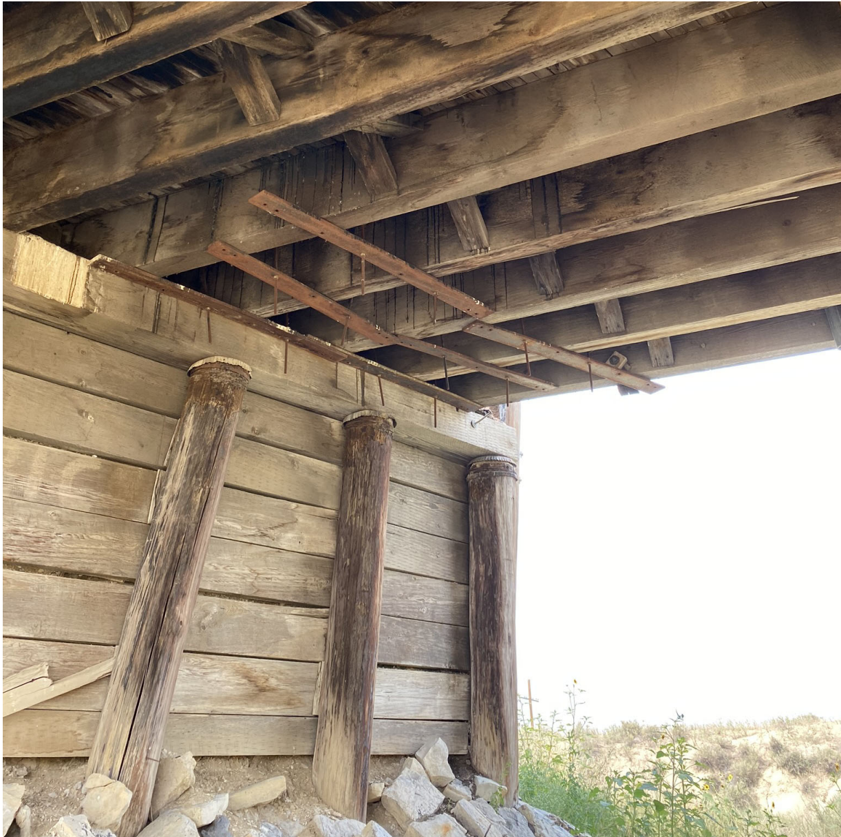
Picture 2 - Repaired Girders
