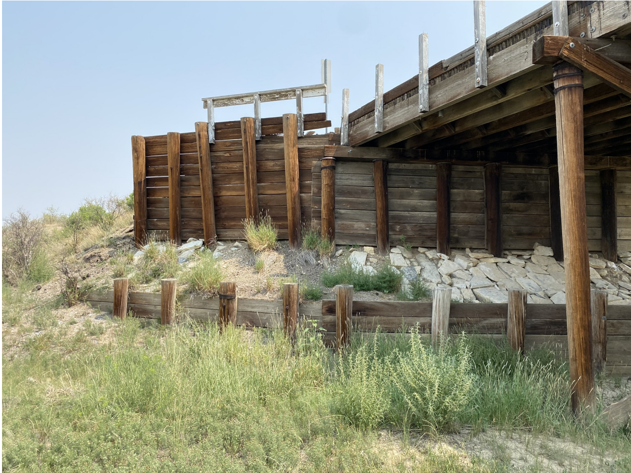
Picture 3 - Girders, Guardrail, Piles
